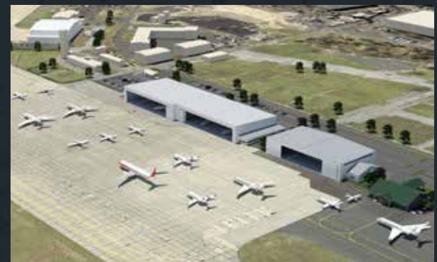
Future New FOK Hangar Complex
